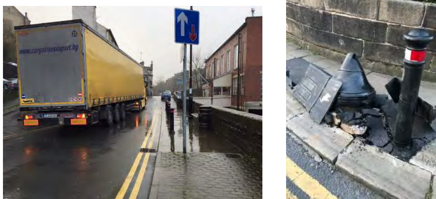
Figure 26 - Truck stuck on Hollowgate, Holmfirth & HGV damage to 'bell' protecting bridge on Hollowgate
