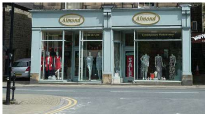
Example of reinstatement of historic-style shopfront.
