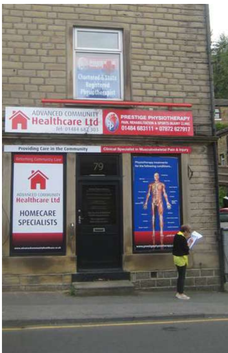
Large fascia and adverts covering three windows.
