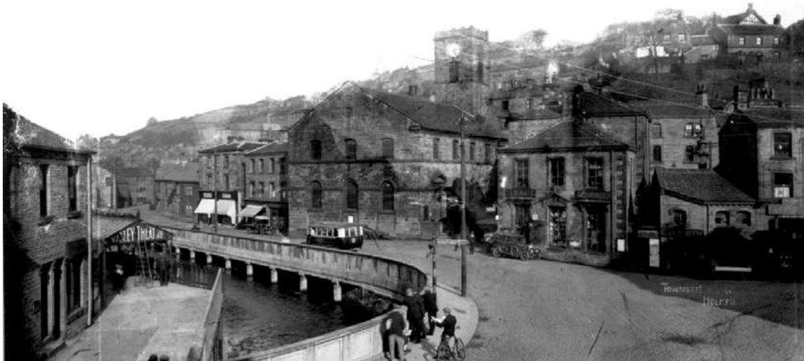
Towngate after demolition showing widened bridge and Victoria Square
