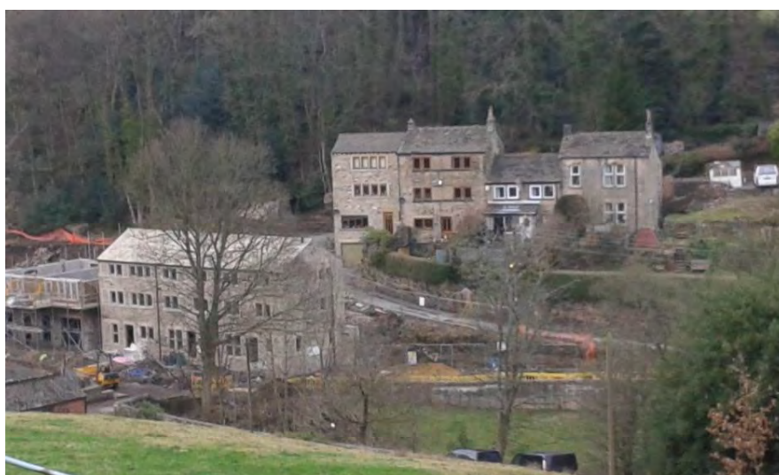
Figure 12 - New build homes being constructed to fit in with the local style, Upperthong
