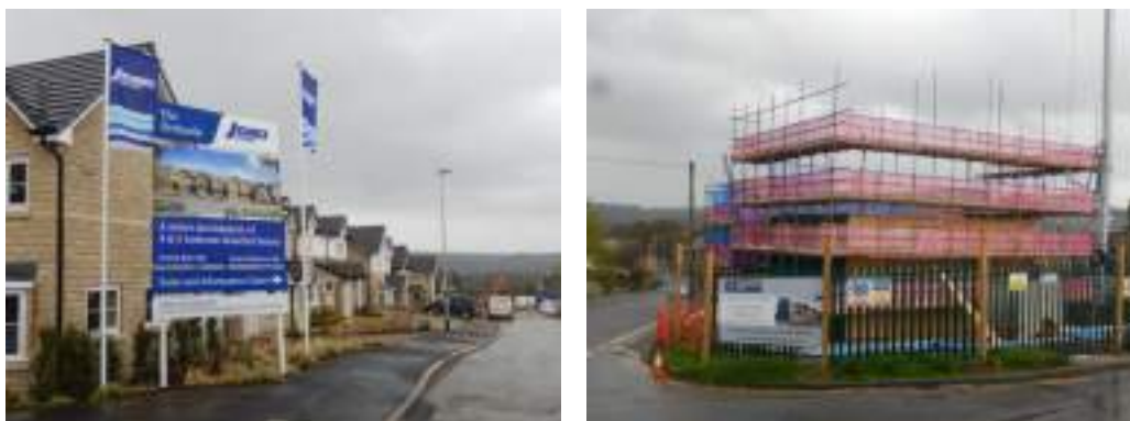
Figure 18 - New developments in Netherthong & Honley
