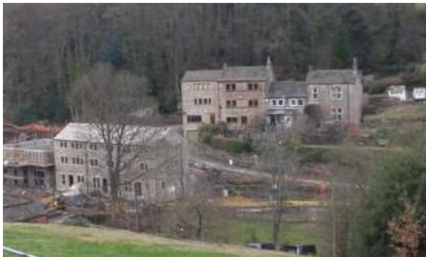
Figure 11 - New build homes being constructed to fit in with the local style, Upperthong
