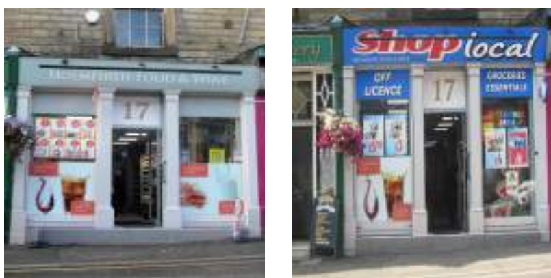
Figure 16 - Recent change of Holmfirth shopfront from traditional to modern design
