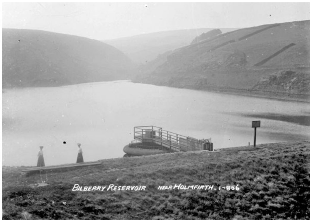
Failure of the embankment walls of the Bilberry Reservoir were responsible for the Great Flood of 1852. Inadequate foundations resulted in cracks and eventual failing of the dam wall which led to flood damage to Holmbridge, Hinchliffe Mill and Holmfirth. Many mill buildings and housing were destroyed and hundreds more were damaged. It also resulted in loss of life.
