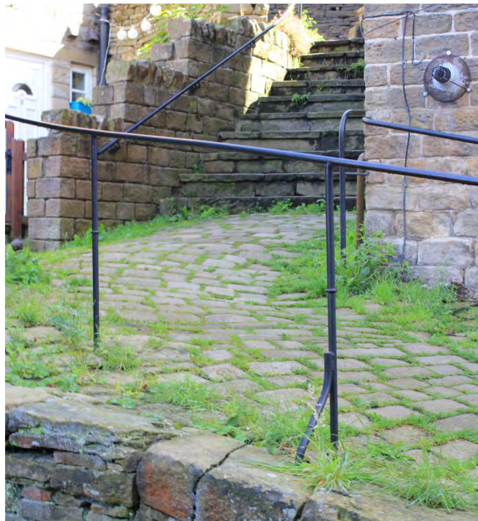
Stone sett paving to the east of Town Gate
