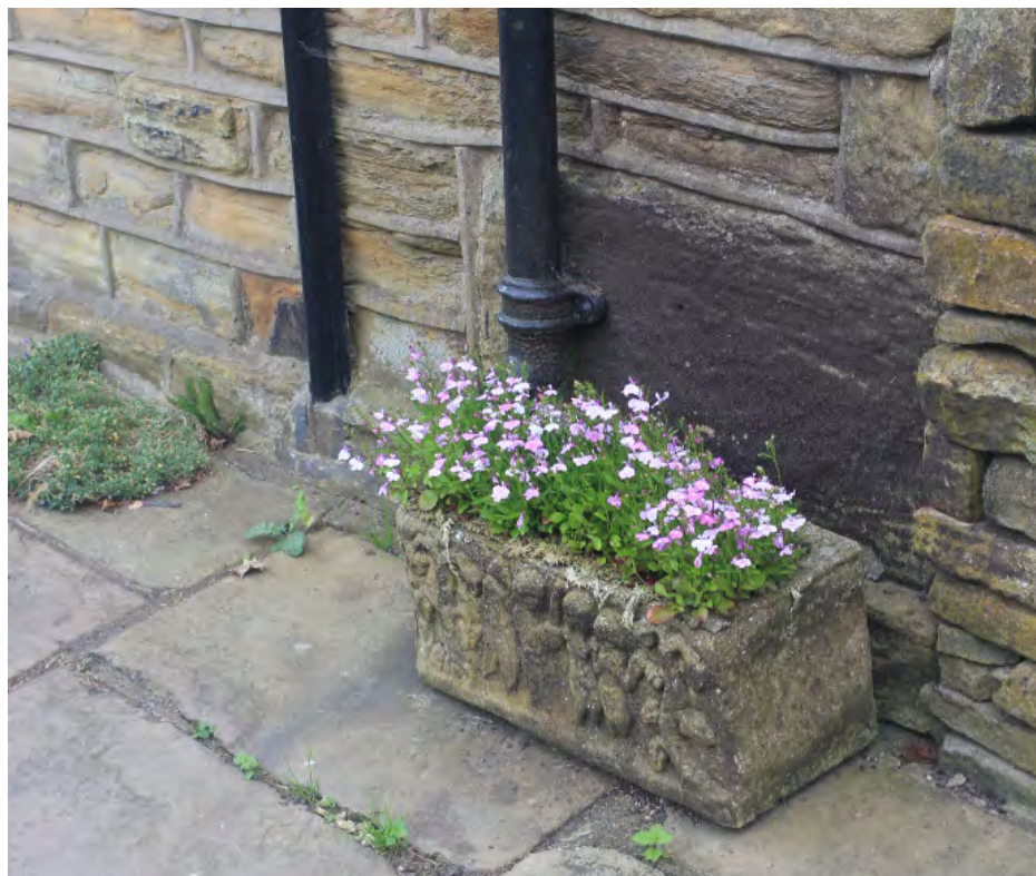
Features within Fulstone Conservation Area
