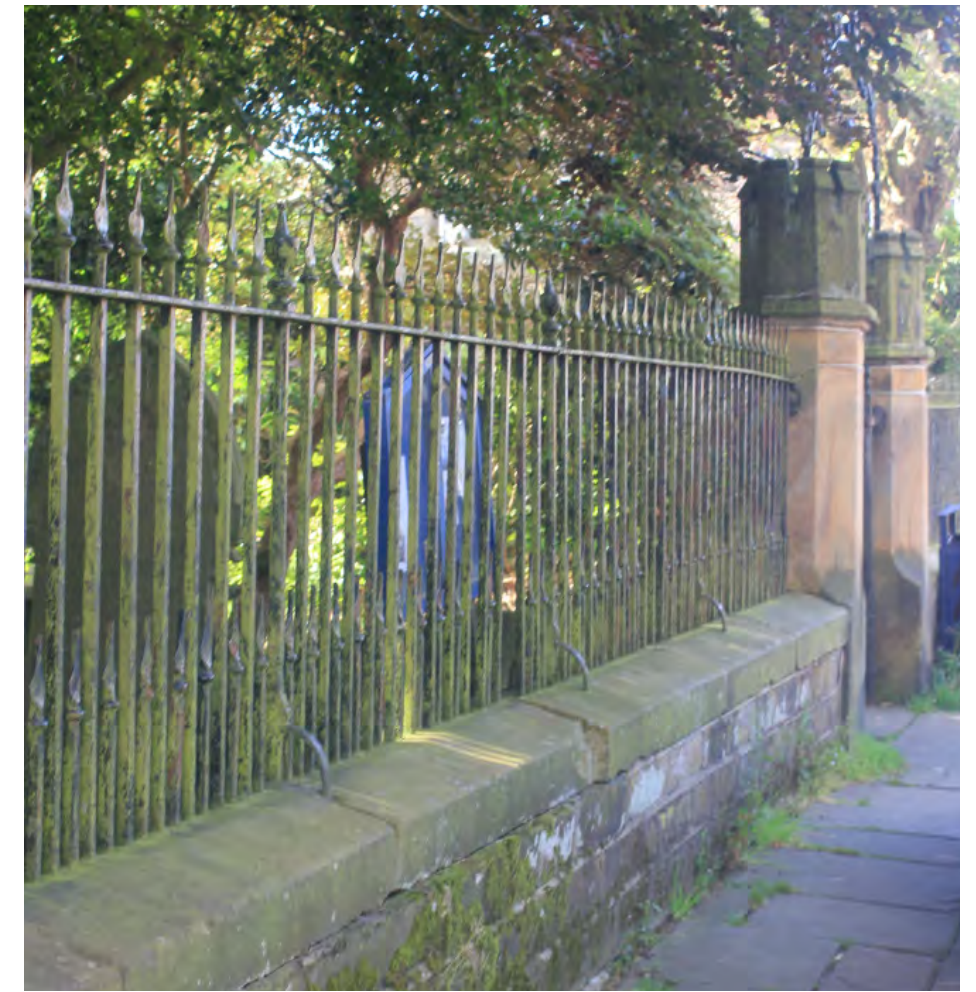
Boundary treatments at All Saints Church, Netherthong
