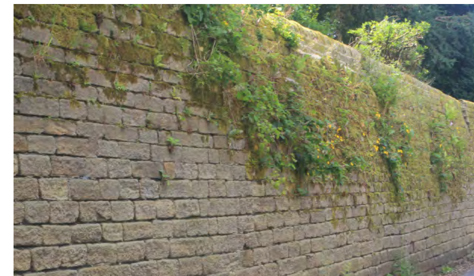
Stone walling parallel Main Gate in Hepworth
