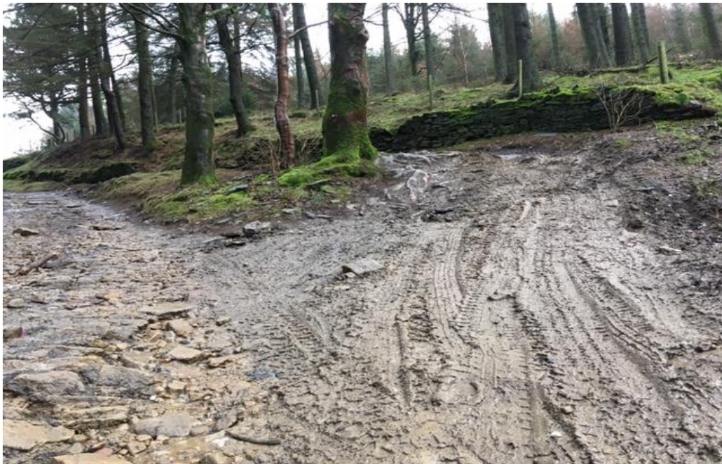
Off road activity on Ramsden Road. The actual route is to the left of the photo but vehicles choose to go around the trees. The roots are now exposed and badly damaged – will undoubtedly lead to the loss of these trees
