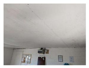
The existing ceiling and exposed electrics prior to the work. Six old fluorescent striplights have been removed to be replaced with more environmentally friendly LED spotlight units to be sunk into the new ceiling, funded by the club.
