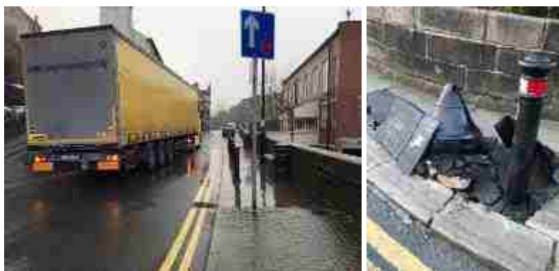
Figure 33 - Truck stuck on Hollowgate, Holmfirth & HGV damage to 'bell' protecting bridge on Hollowgate
