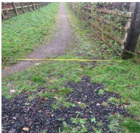
PHOTO 3: Around 90-degree left turn looking westwards = 2.10m at narrowest point to grass banking
