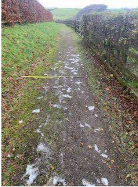
PHOTO 4: Moving from Point A towards Point C around first sweeping bend from west to north/northwest = 2.40m fence to grass banking
