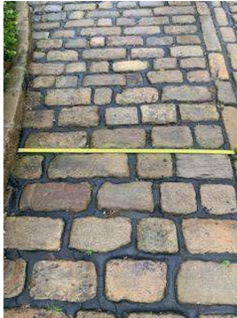
PHOTO 10: Surface at Point C on the Order Plan as the Diversion Route meets Wolfstones Road = 1.20m width from low planter to vertical cobble setts on adjacent driveway
