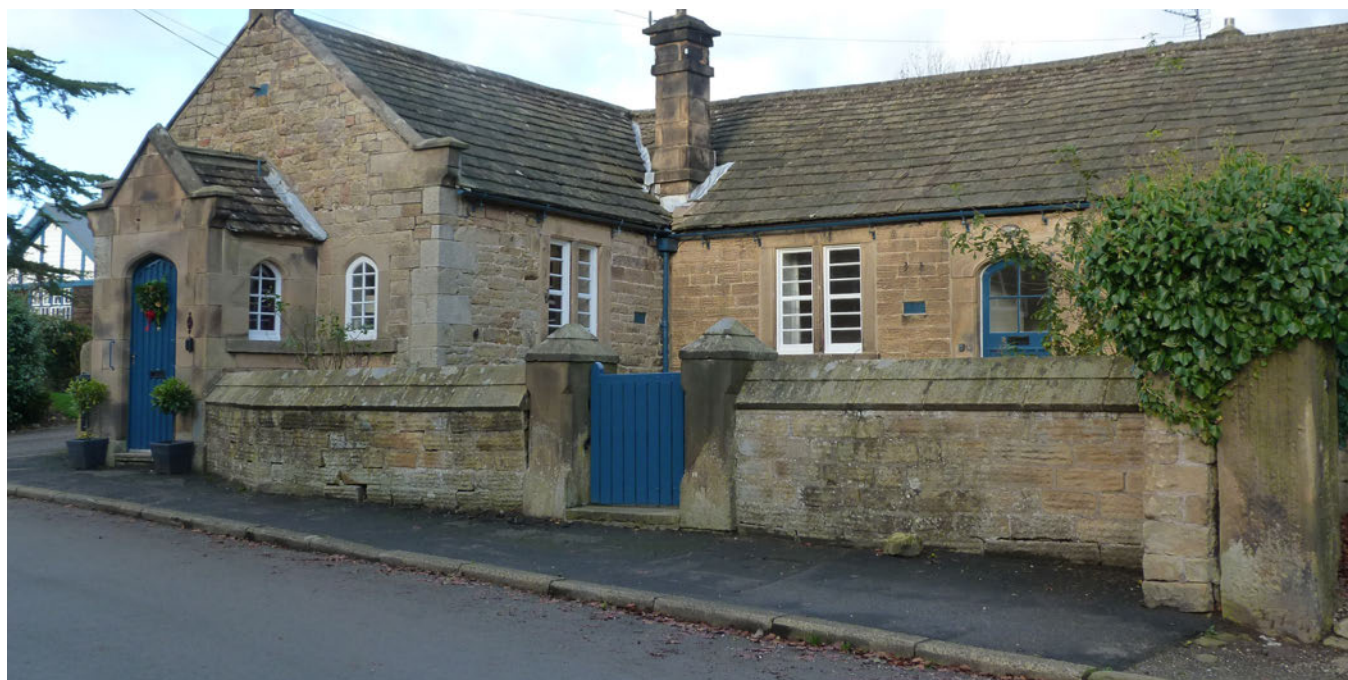
This former school is now a domestic dwelling, but retains its institutional character. (© PDNPA)
