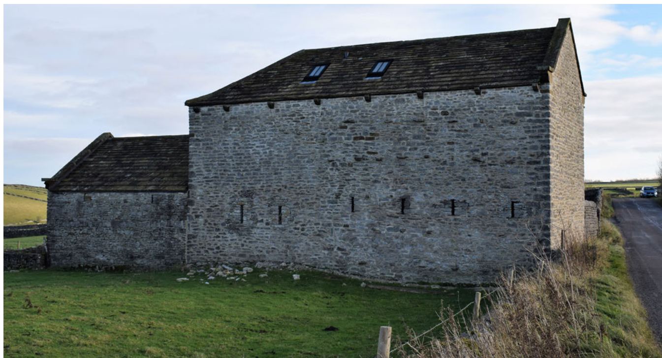
A barn after conversion – the solid-to-void ratio has been maintained. The only alterations on this elevation are two conservation rooflights and two additional vent slits to allow additional light to the interior. All the other original openings are on the opposite elevation. (© PDNPA)
