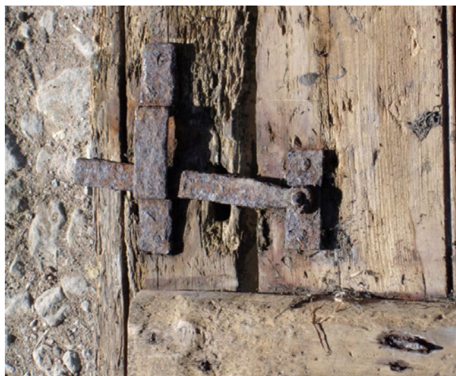
A simple iron latch on a historic door. (© PDNPA)
